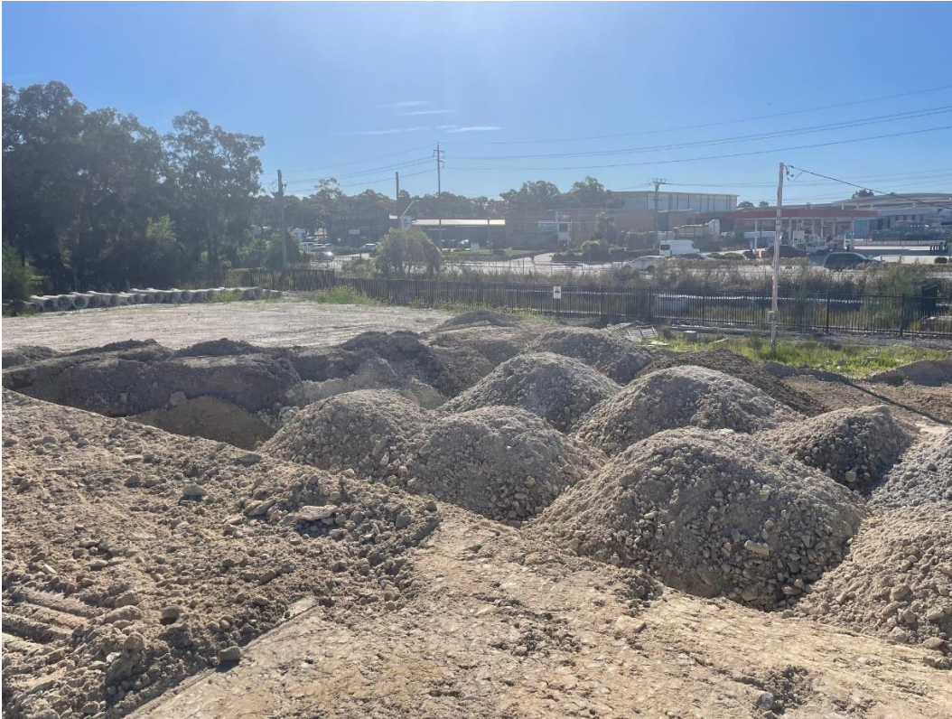
Photograph 3.1 North-west corner of the site
